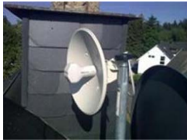
Figure 12: Typical BFWA TS antenna (Ubiquiti Networks, www.ubnt.com )
