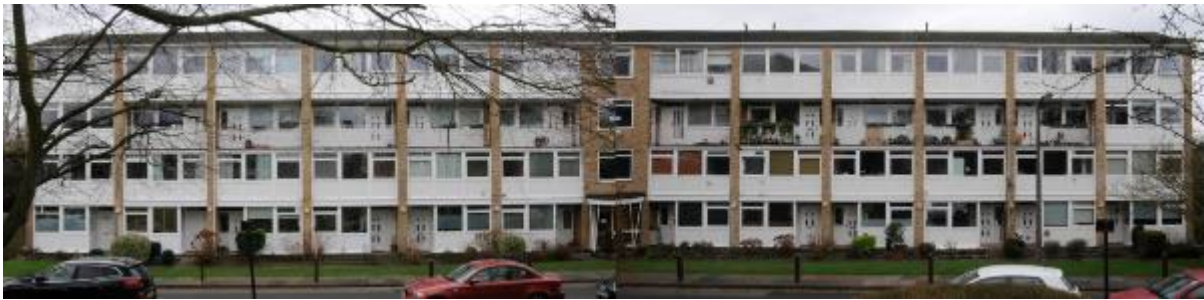
Figure 26: Apartment block in Southeast London
