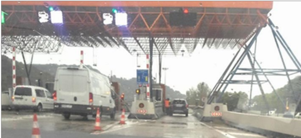
Figure 3: Toll plaza on the Spanish motorway C-32
