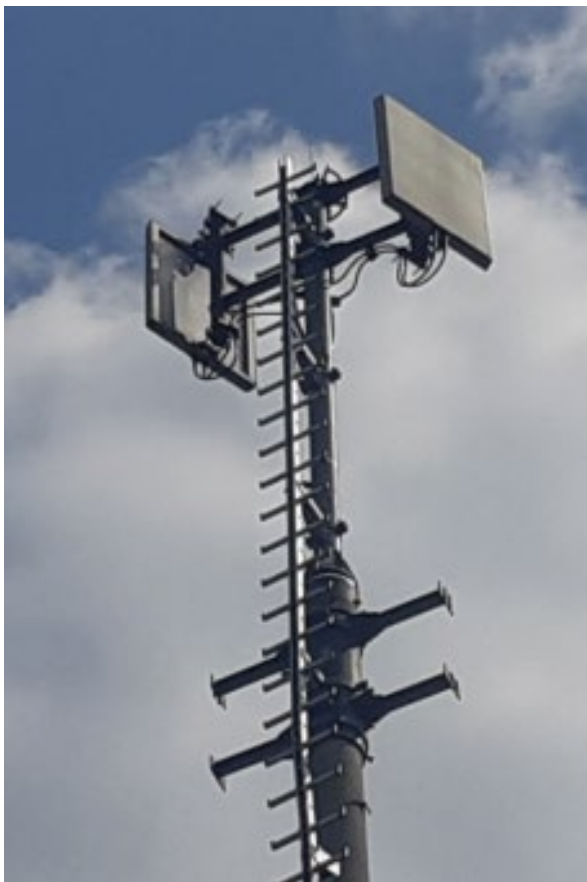
Figure 59: Typical RMR (left) and MFCN (right) antenna installations
