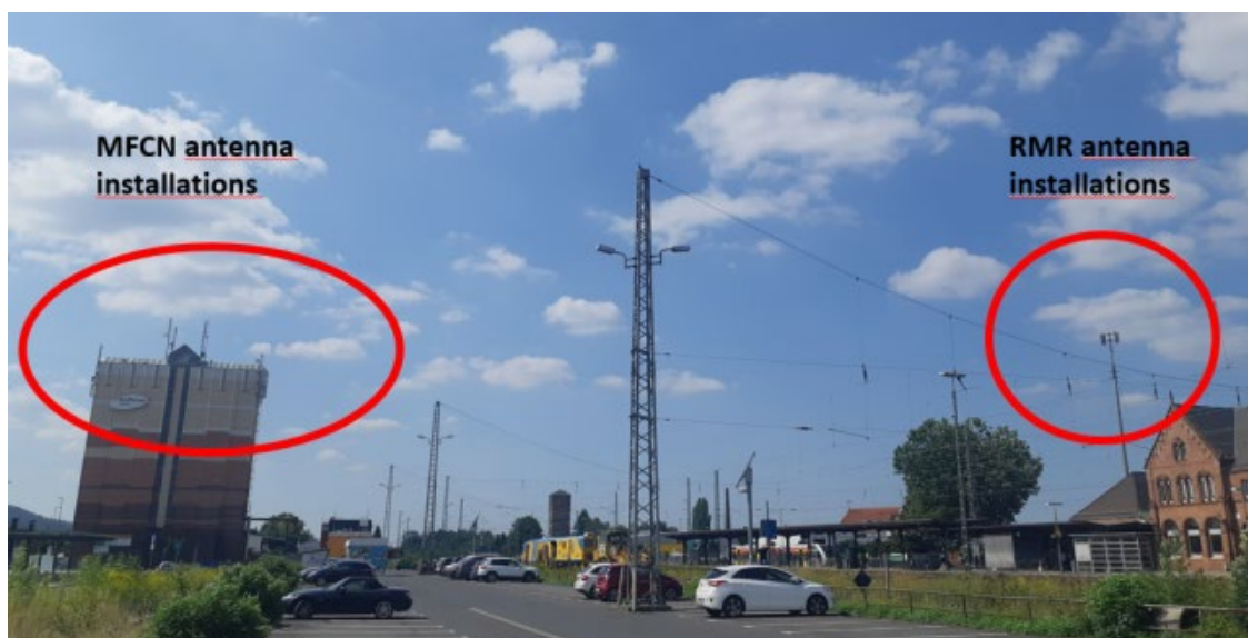
Figure 63: Typical scenario of RMR and MFCN antenna installations
