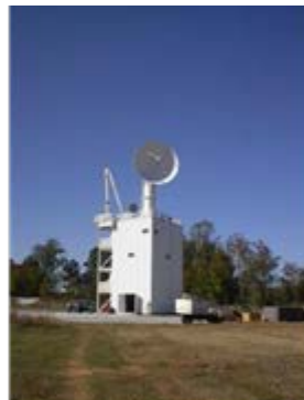
Jackson County Pattern Range Receive Tower and Control Room
