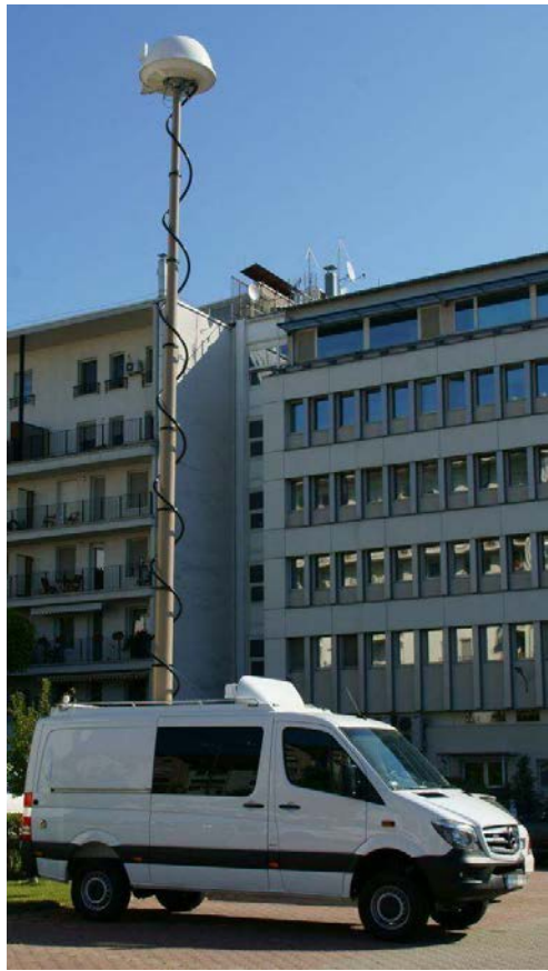
Figure 10: DF and monitoring antennas fixed on the top of the mast (Hungary)
