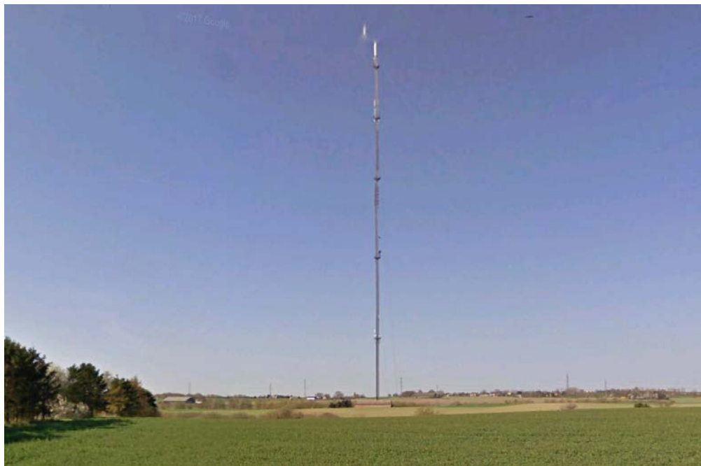
Figure 187: LTE 450 MHz main site for Copenhagen (image source google maps)
