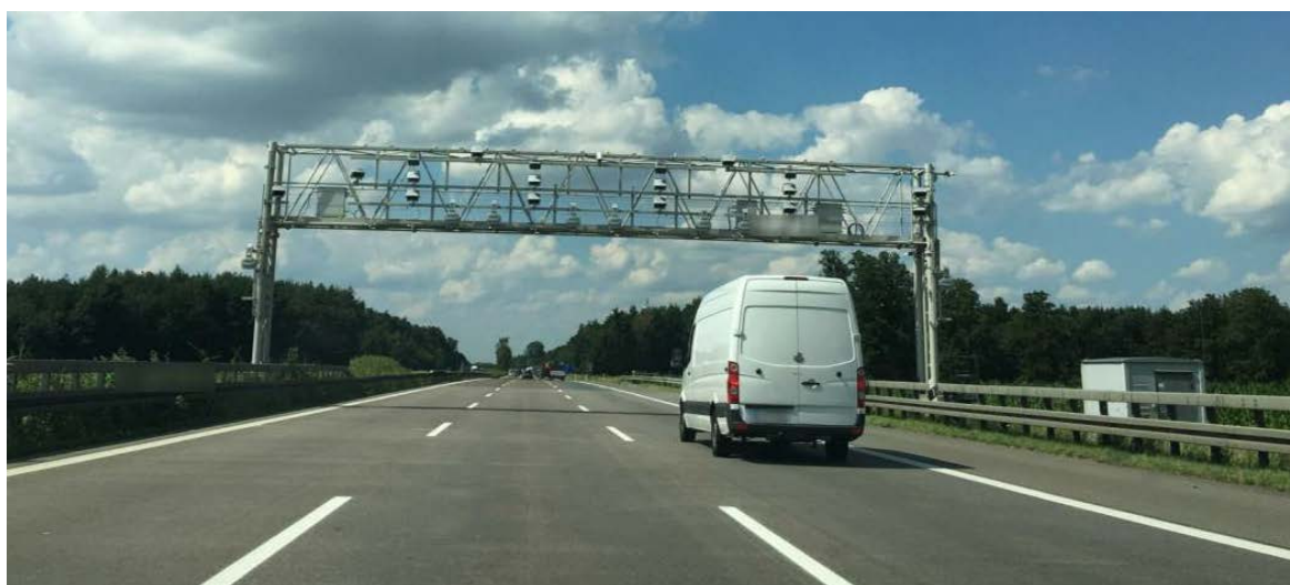
Figure 18: DSRC Gantry on the German motorway A9
