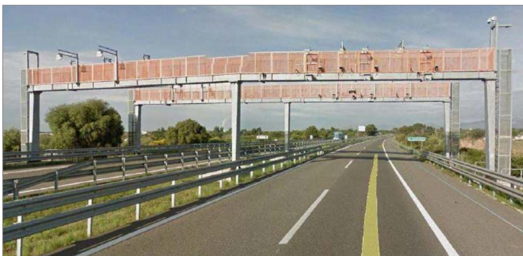
Figure 16: Toll gantry on the Spanish motorway AP-7
