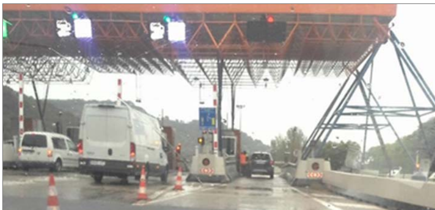
Figure 15: Toll plaza on the Spanish motorway C-32
