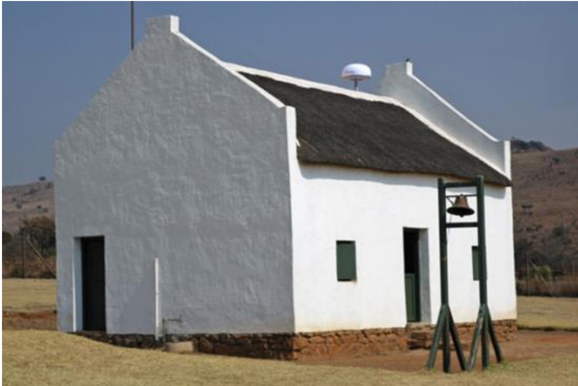
Figure 7: Example of parabolic antenna
