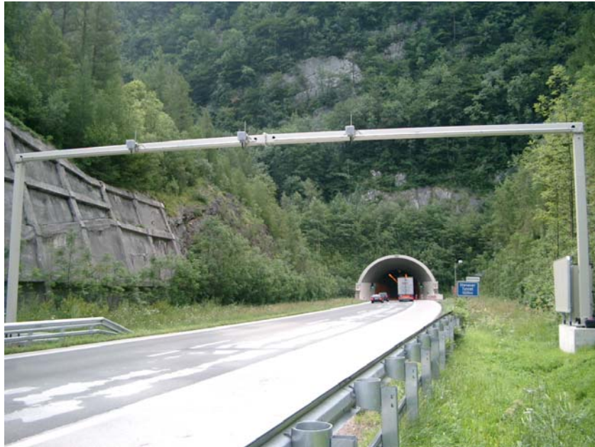
Figure 8: Typical free-flow installation with three lanes
