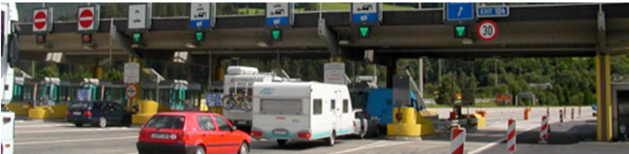
Figure 9: Typical toll plaza with an automatic barrier (left) and a single automatic lane (right)
