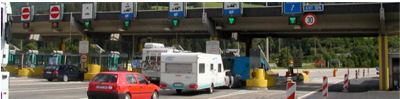
Figure 11: Typical toll plaza with an automatic barrier (left) and a single automatic lane (right)
